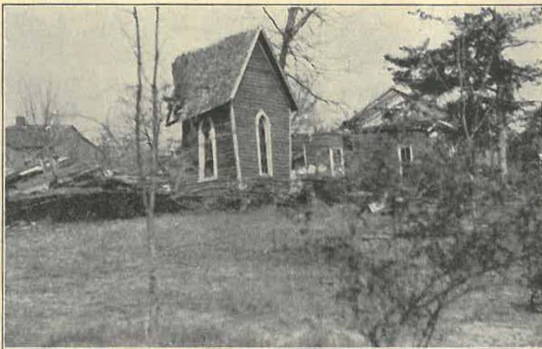
AFTER THE TORNADO
