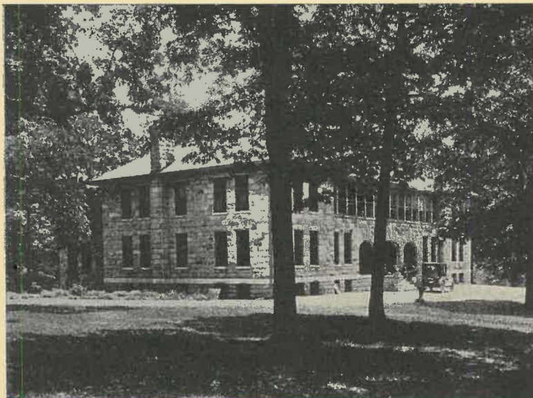
EMERALD HODGSON HOSPITAL, SEWANEE, TENN.
