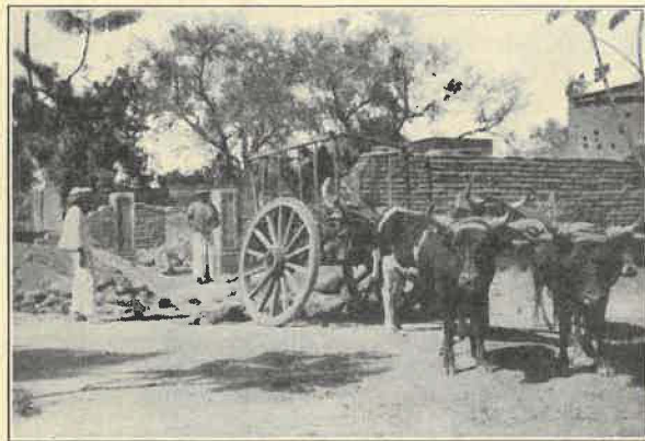
AT SAN SEBASTIAN Building the new church at San Sebastian, Jalisco.
