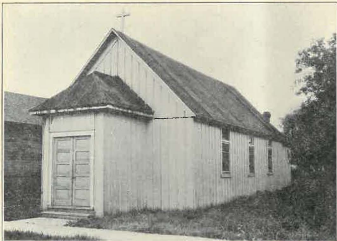
OLD ST. LUKE'S, RENTON, WASH.
