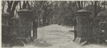
An Historic School in an Historic City
