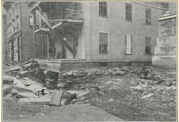
FLOOD DAMAGE TO CHRIST CHURCH PARISH HOUSE
