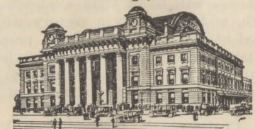
Chicago Passenger Terminal 762
