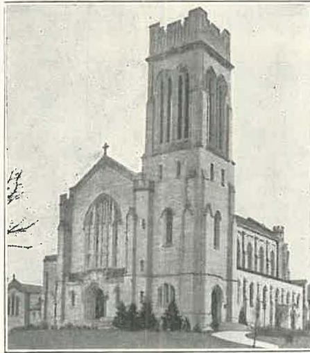
ST. MARK'S CHURCH, MINNEAPOLIS, MINN.
