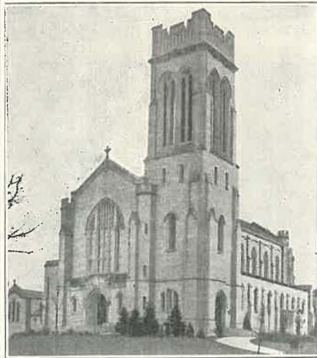
ST. MARK'S CHURCH, MINNEAPOLIS, MINN.
