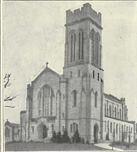
ST. MARK'S CHURCH, MINNEAPOLIS, MINN.
