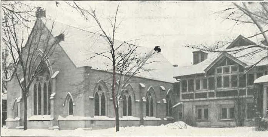
CHRIST CHURCH AND PARISH HOUSE, EAU CLAIRE, WIS.
