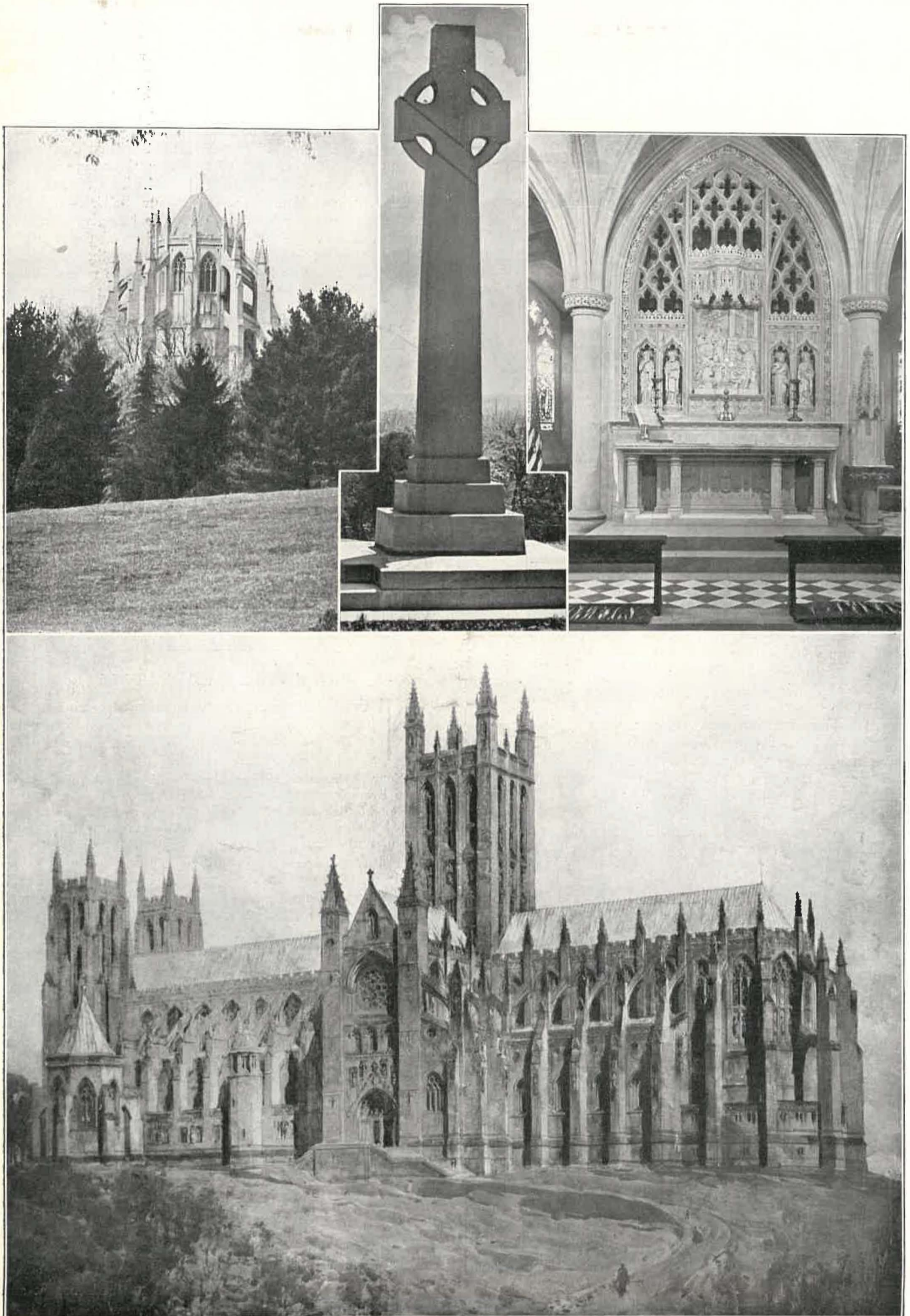
VIEWS OF THE WASHINGTON CATHEDRAL ABOVE, AT LEFT: THE APSE, SEEN FROM WOODLEY ROAD. AT CENTER: THE PEACE CROSS. AT RIGHT: ALTAR AND REREDOS IN THE BETHLEHEM CHAPEL. THE CRYPT. BELOW: WASHINGTON CATHEDRAL, WHEN COMPLETED: VIEW FROM THE SOUTHWEST. [From the Architects' Drawing]
