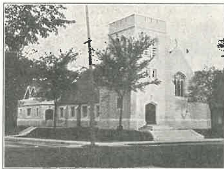
ST. JOHN'S CHURCH, LINDEN HILLS, MINNEAPOLIS, MINN.
