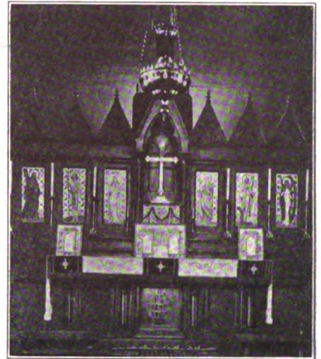
ALTAR AND NEW PANELS IN ST. JAMES' CHURCH, CLEVELAND, OHIO
