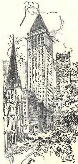
Bankers Trust Company Building
