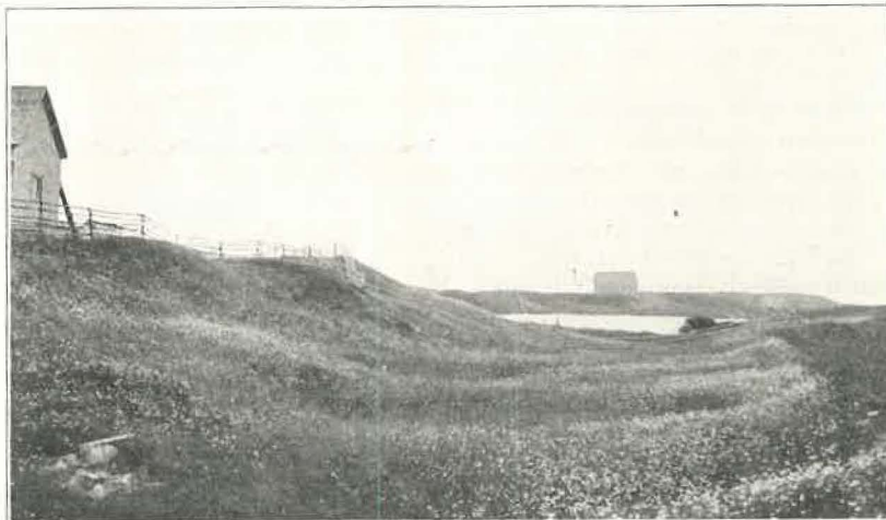
EARTHWORKS AT LOUISBOURG
