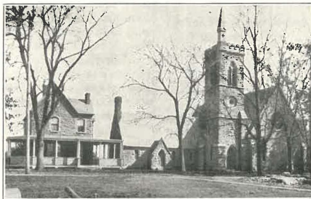
ST. JOHN'S CHURCH, MONTICELLO, N. Y.
