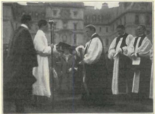
AT THE BREAKING OF THE GROUND FOR THE NAVE OF THE CATHEDRAL
