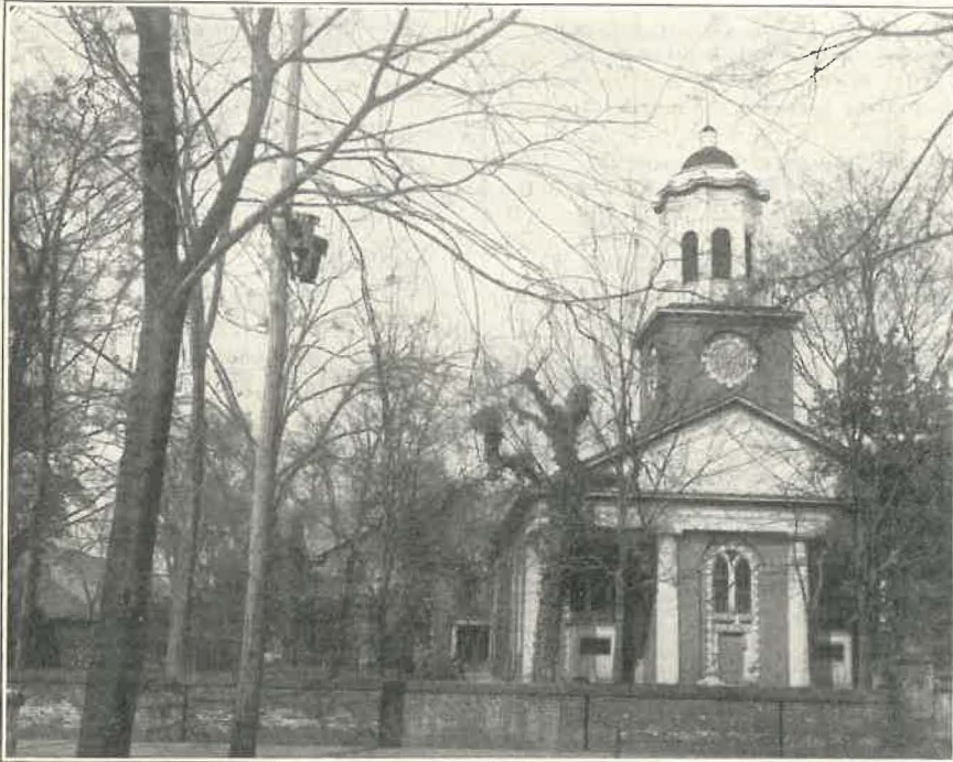
ST. PAUL'S CHURCH AND PARISH HOUSE, AUGUSTA, GA. Historic colonial building destroyed in the great fire of March 22, 1916 [See LIVING CHURCH of April 8, p. 825]
