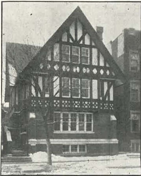
RECTORY, CHURCH OF THE REDEEMER, CHICAGO
