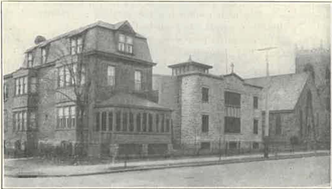
GROUP OF BUILDINGS OF ST. GEORGE'S CHURCH West Philadelphia
