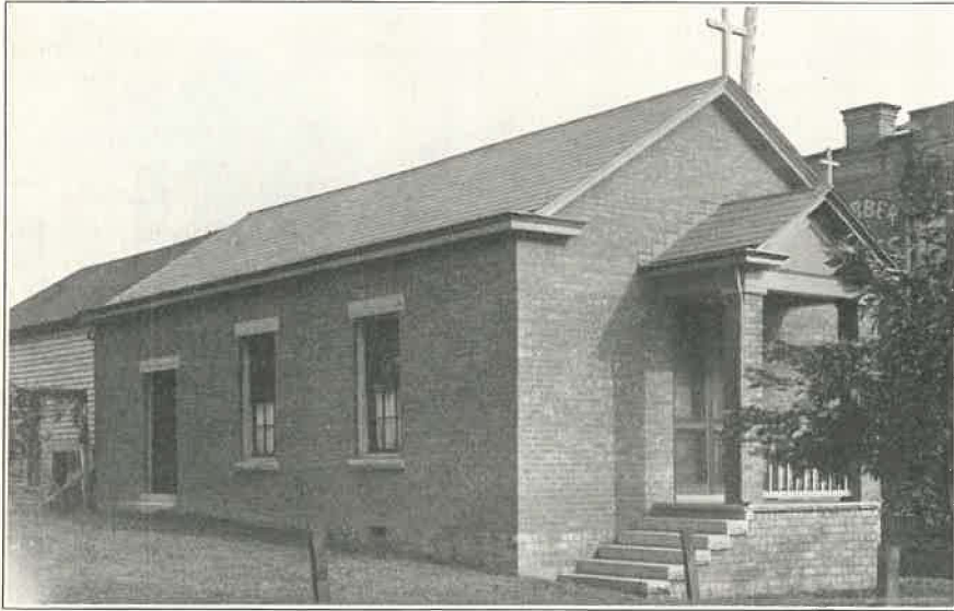
PARISH HOUSE OF CALVARY CHURCH, ASHLAND, KY.
