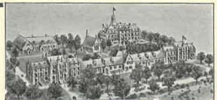
View of the School Buildings
