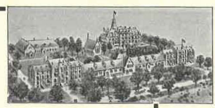
View of the School Buildings
