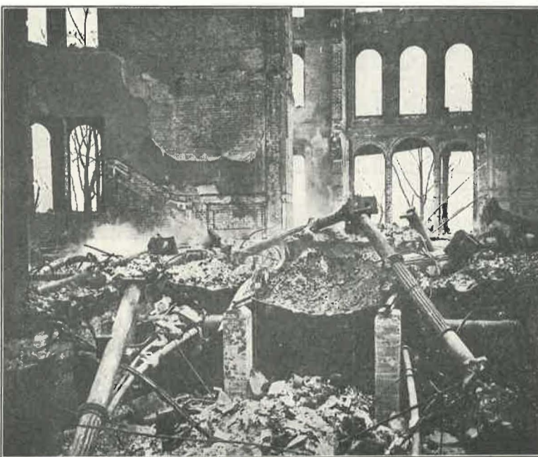
"THE CENTRE," COLLEGE HALL AFTER THE FIRE. WELLESLEY COLLEGE
