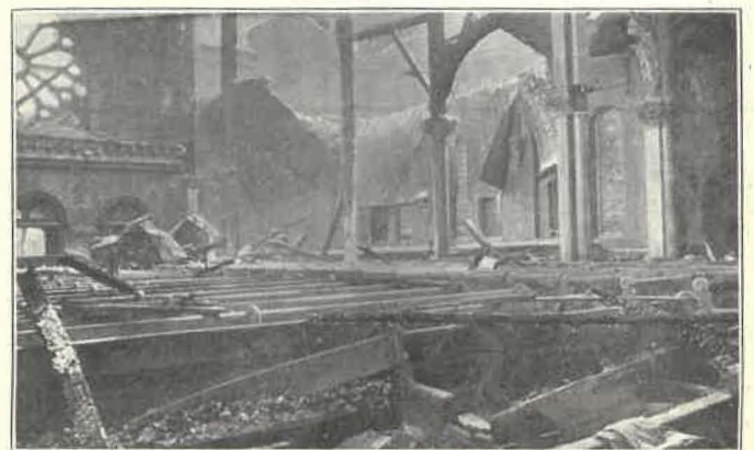
WHERE THE DAMAGE WAS GREATEST. SUNDAY SCHOOL BUILDING IN BACKGROUND
