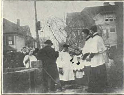
LAYING THE CORNERSTONE St. Jude's, Brooklyn
