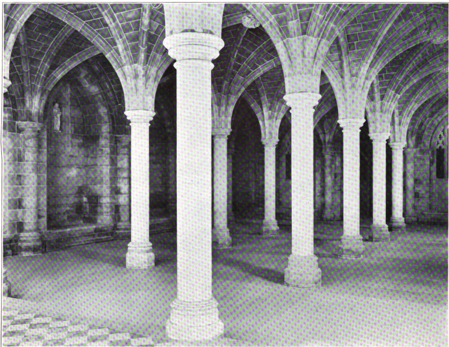
THE NAVE FROM THE CHANCEL
