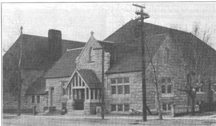
NEW PARISH HOUSE OF ST. MARK'S CHURCH, CHEYENNE, WYO.
