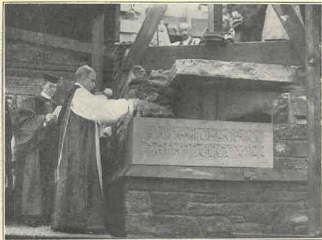
LAYING THE CORNERSTONE, INTERCESSION CHAPEL, NEW YORK [Showing Bishop Greer and the Architect, B. G. Goodhue, of the firm of Cram, Goodhue & Ferguson]
