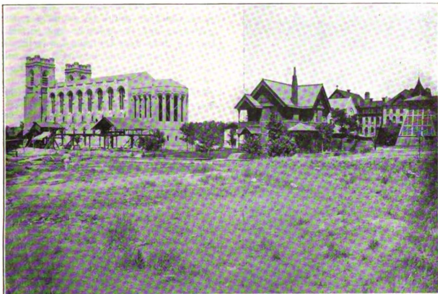
CATHEDRAL OF ST. JOHN THE EVANGELIST, DENVER—IN COURSE OF ERECTION.
