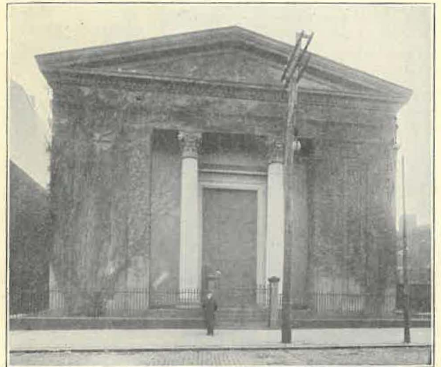
OLD TRINITY CHURCH, Southwark, Philadelphia, now to be demolished.
