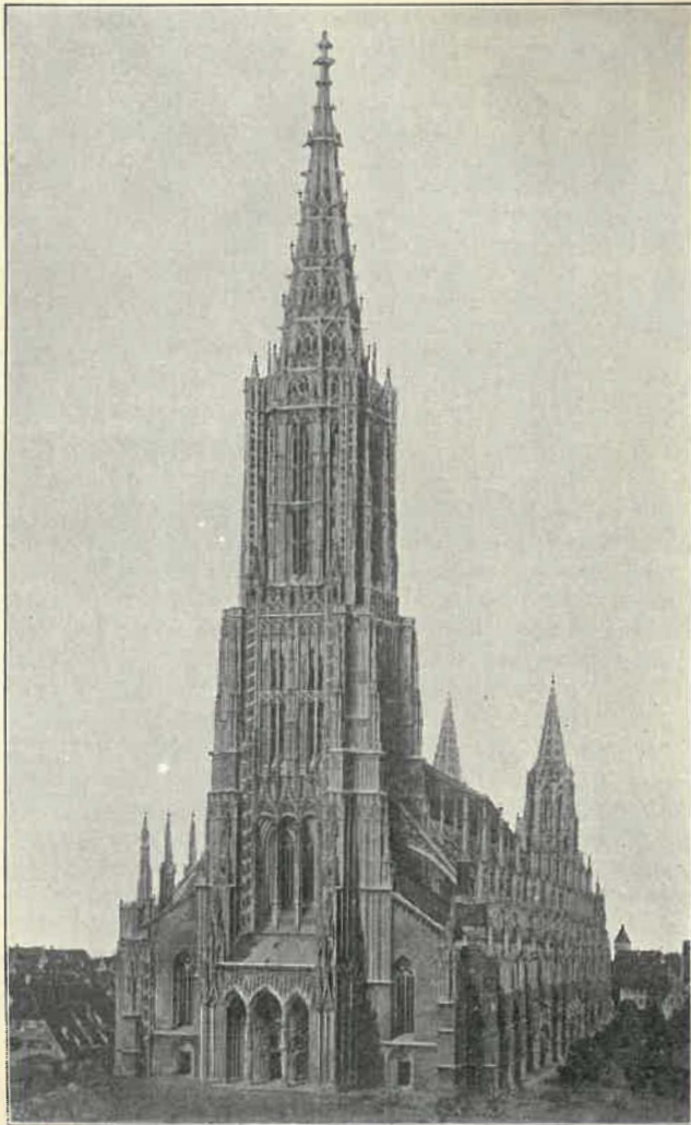
MINSTER OF ULM—FACADE AND TOWER.
