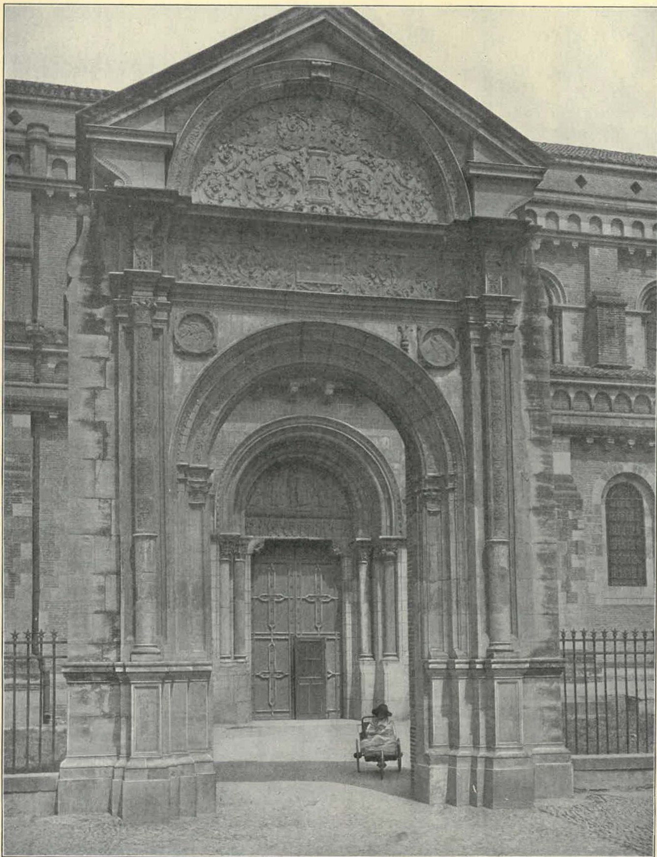
ST. SERVIN, TOULOUSE--SOUTH PORTAL.
