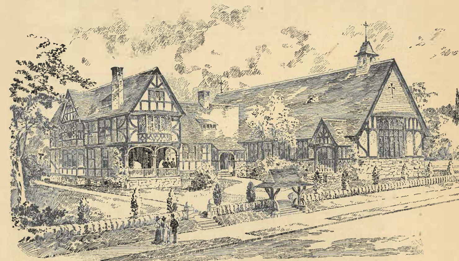
ST. PHILIP'S CHURCH AND RECTORY, DYKER HEIGHTS, BROOKLYN.
