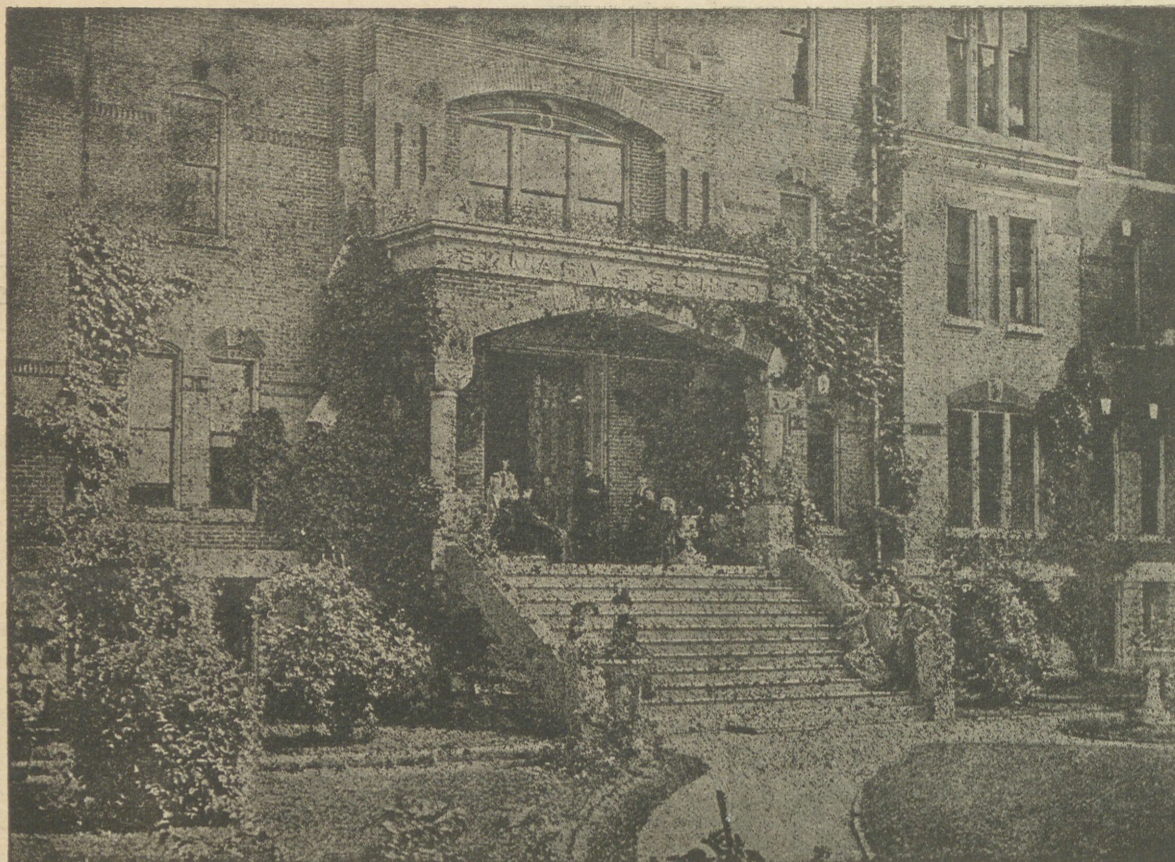
MAIN ENTRANCE TO ST. MARY'S SCHOOL, KNOXVILLE, ILLINOIS.
