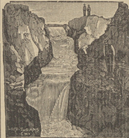
OVERFLOW OF CANAL—60 ft. FALL.
